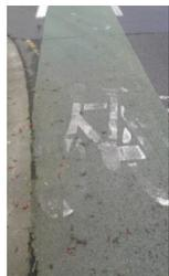
One major issue is surface color and paint can fade. If the surface material is integral to the asphalt mix (red in the Netherlands), the color won't wear off as with paint. If a bicycle symbol is painted, it will wear off faster than a bike stencil in preformed thermoplastic but those, especially in wet weather, can be slippery.
