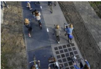
Solar panels have been embedded into a cycle path in the Netherlands for a length of 230 feet. Though viewed pessimistically because the panels on the flat surface were not pitched toward the sun and shadows from bicyclists and trees would lessen the energy generated, the solar panel cycle track has generated power. Time will tell if maintenance issues are complex and costly.
