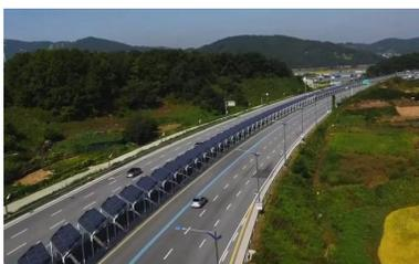
In locations where rain is constant or sun unrelenting, perhaps the solar panels could be elevated like a carport, tilted toward the sun but also with a continuous roof to protect from rain and snow. This would resemble the full sidewalk-width storefront canopies in early American small towns and in Australia to shade patrons. This solar covered cycle track could be in a location that is not in the middle of a major highway.
