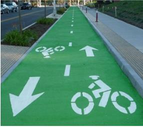
To designate a road or cycle track area as being for bicyclists, sometimes the pavement is of a different color. One option is to put a pigment into the pavement, as in the red pavement in the Netherlands. Another option is to paint the surface of the asphalt but this can wear off or be slippery. A new option is the product by Transpo Industries. The material is applied to the surface of the asphalt and comes in a variety of colors.
