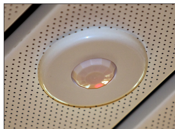
Among the new sustainability features at Rockefeller Hall are a motion detector on the cafeteria ceiling (left) that is linked to an air handler unit; energy-saving, motion-activated faucets (above left); double-paned windows (top) that contain a gas that filters out excess sunlight in hot months; large, easy-to-access recycle areas (above); and a carbon dioxide sensor (right) on the wall of the cafeteria that activates fans depending on the number of people in the room.
